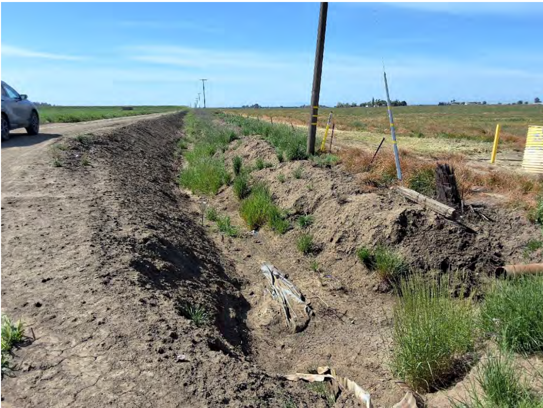
Site access off Tremont Road showing Solano Irrigation District's canal, with a sidewall that was recently scraped to remove vegetation.
