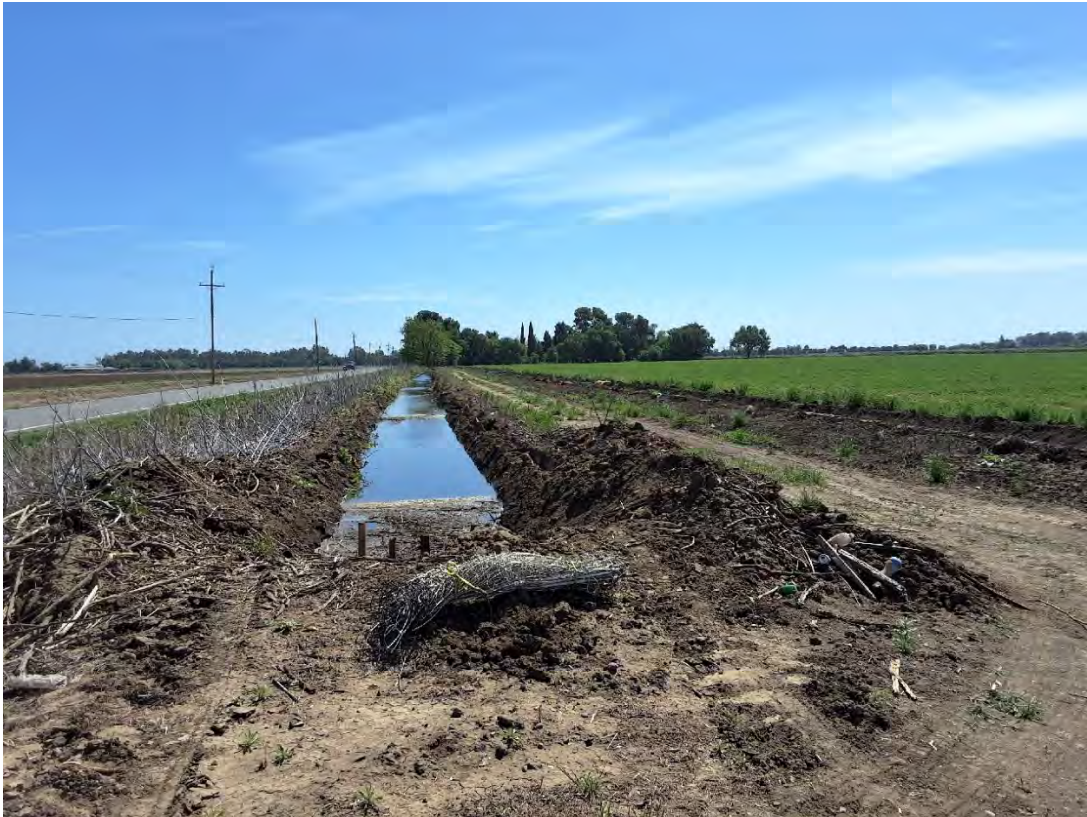
Irrigation ditch parallel to Tremont Road that is filled by groundwater pumped from a well.
