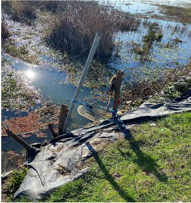
Photograph 5. The out fall culvert from Watson Hollow Slough and in-fall culvert to the wide ditch have gate valves which are operable and are located at the north end of the ditch.
