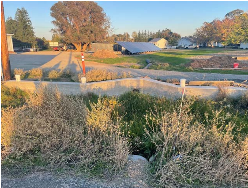
Concrete Wall and Culverts
