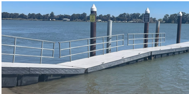
Figure 5/6 Punctured dock floats causing the dock to sag and lose buoyancy
